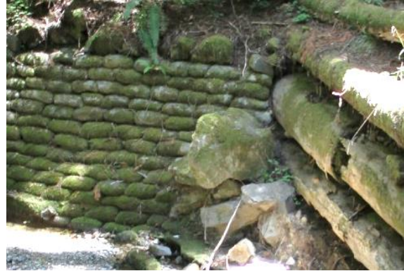
Erosion control efforts in Fife Creek
