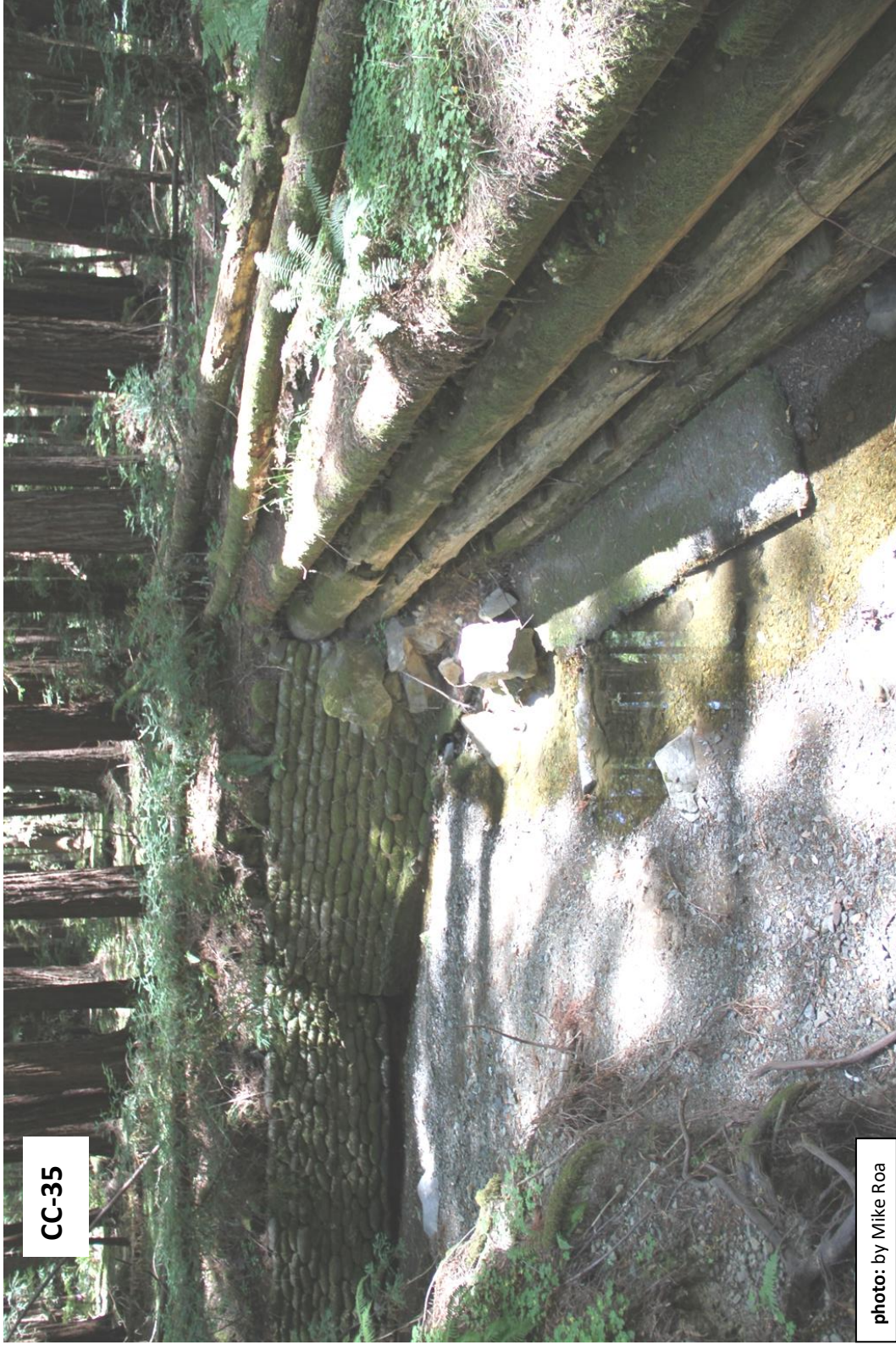
Logs, bags of concrete, and concrete slabs were used to try to control the flow of Fife Creek so that it wouldn't undercut the road and trees. (after 1964 northern Ca floods) Unfortunately, such creek modification damages fish habitat.
