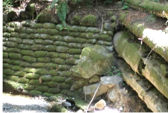
Erosion control efforts in Fife Creek
